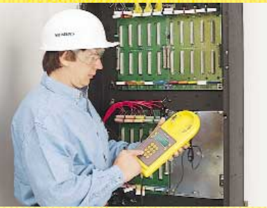
Hand-held Device Programmer and Loop Tester helps reduce installation time.
